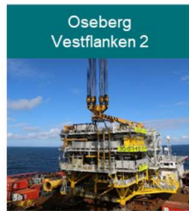
Unmanned Wellhead Platform (UWP™)
