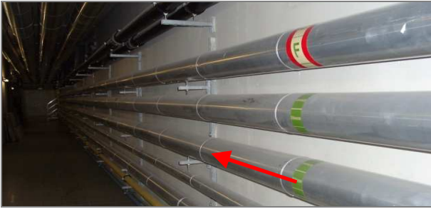
Fig. 4. Photography of an outstretched utility corridor.
