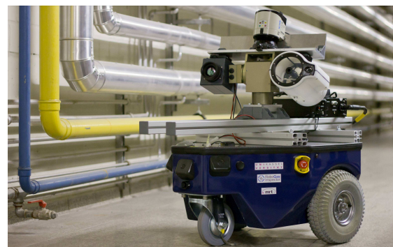
Fig. 10. Lab inspection robot with first-gen. sensor head.
