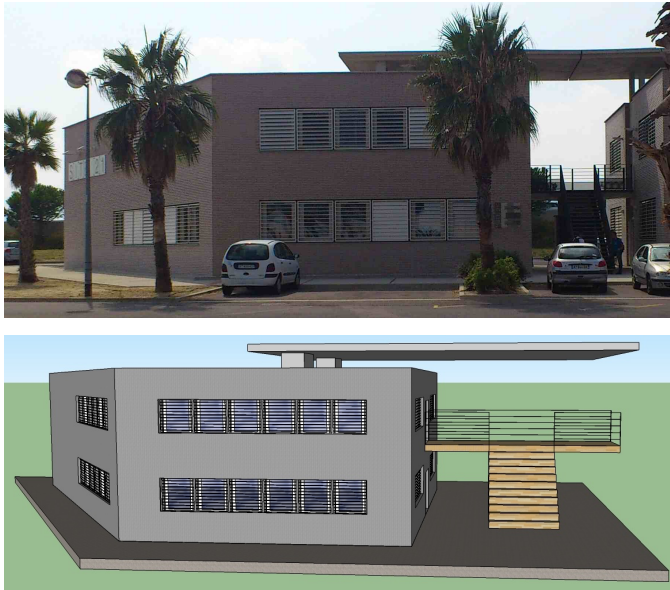
Fig. 1. Photography of the two floors building under study and the corresponding Google Sketchup mock-up.
