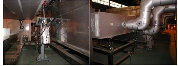
Fig. 3. The pyrometer and thermocouples installed on the inductive heating oven
