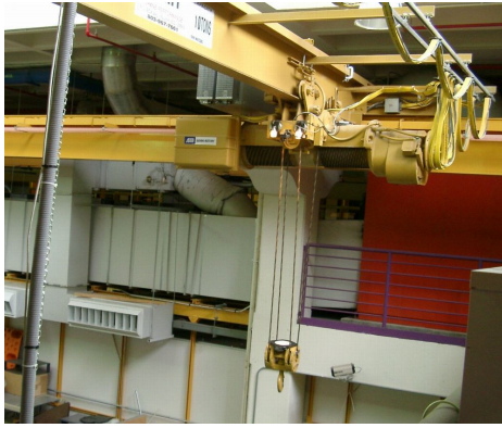
Fig. 3. 10-Ton Bridge Crane at Georgia Tech shaping is enabled. The two responses are from the same human operator. The figure shows that under normal operation the payload has large oscillations. These oscillations are virtually eliminated by input shaping. Such dramatic performance improvement motivates students to understand the control system, especially when they are the ones driving the crane. Input shaping also proves a worthwhile contrast to the feedback methods taught in controls coursework and allows illustrative comparisons between open and closed-loop control methods.
