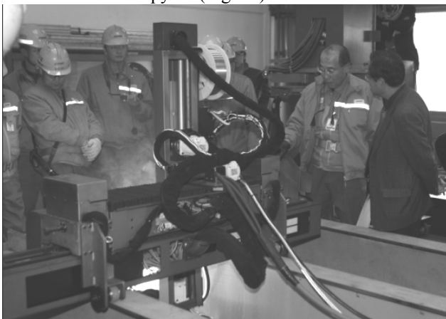
Fig. 11. Validation of welding task of RRX3
