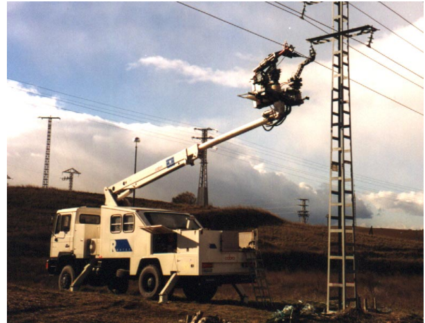
Fig. 2 Insulator set change by the ROBTET
