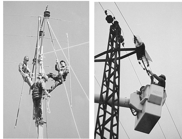
Fig. 1 Indirect work (using hot-sticks) and direct work (from a bucket)
