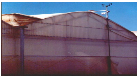
Fig. 1. Detail of the Araba greenhouse
