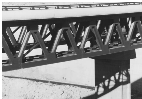
Fig. 1. Inspection environment for climbing robot.
