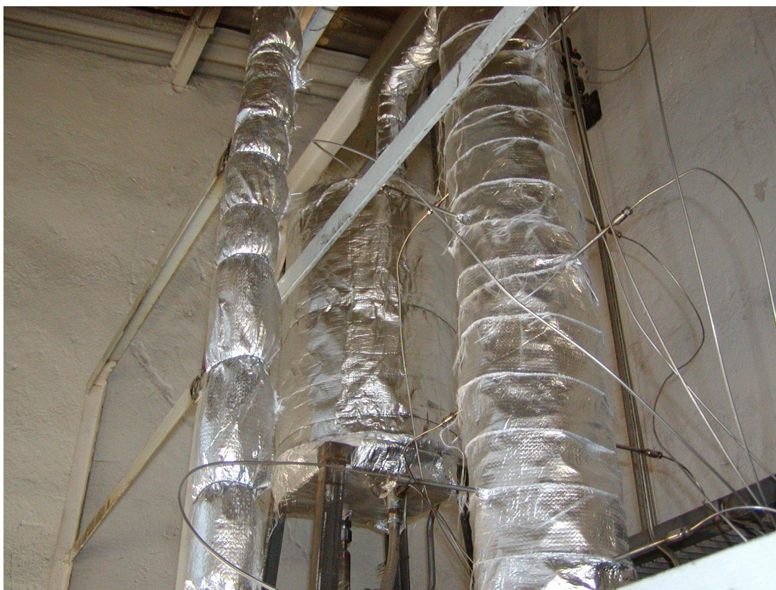
Fig. 1. Photo of insulated pilot trickle bed reactor with set of thermocouples.
