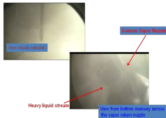
Figure 5. View inside Kettle with C6/C7 system at 38 kW/m 2 Heat Flux
