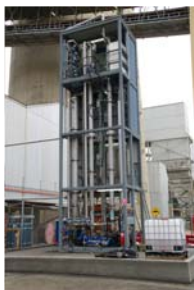
Figure 2: CSIRO pilot plants in Australia. Left: PCC pilot plant at Loy Yang Power based on amines. Right PCC pilot plant at Delta Electricity Munmorah Power station based on aqueous ammonia.
