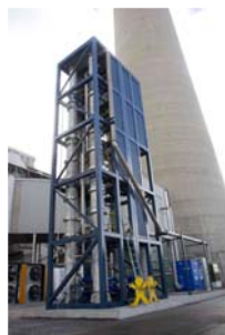
Figure 2: CSIRO pilot plants in Australia. Left: PCC pilot plant at Loy Yang Power based on amines. Right PCC pilot plant at Delta Electricity Munmorah Power station based on aqueous ammonia.
