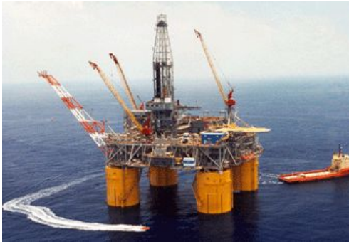
Figure 13. A typical TLP facility
