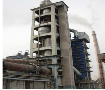
Fig. 6. Scene of raw meal calcination process in the plant
