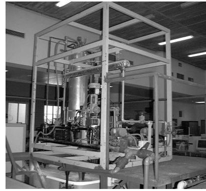
Fig. 1. Pilot plant used to apply the MMMPC.
