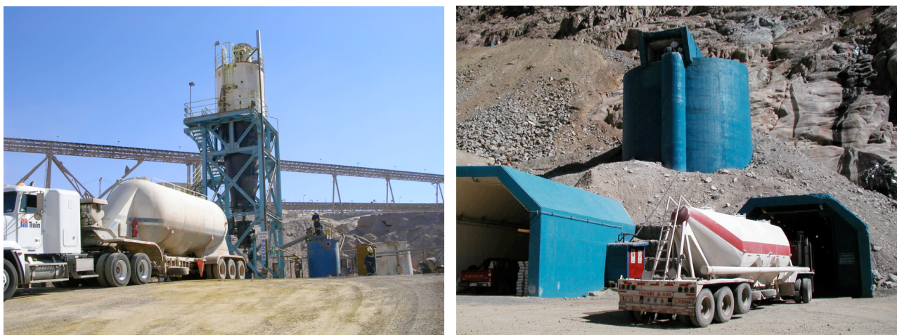
Figure 1: Examples of two Chilean applications with PD trucks ready to unload lime. [3]
