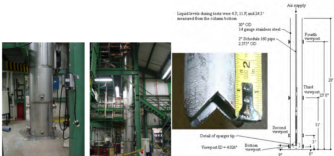
Figure 3: Bubble Column Design and Installation 1
