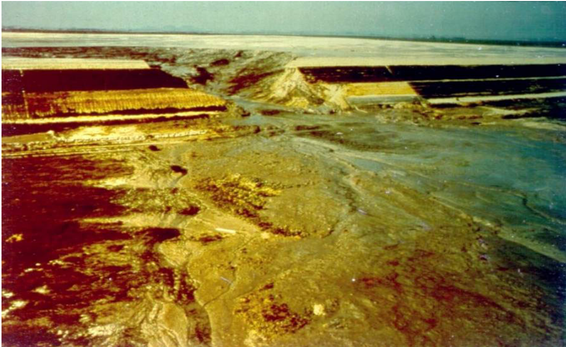
Figure 1: Failure of the Boliden lead-zinc tailings dam in 1998.
