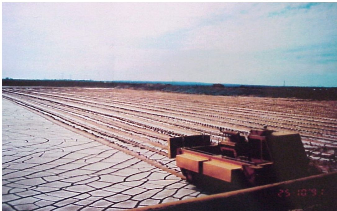
Figure 3: Alcoa Western Australia, bauxite waste dry stacking.
