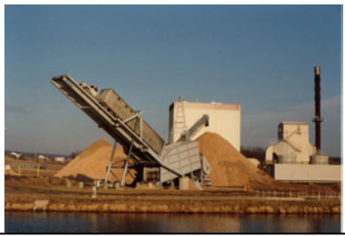
Unloading wood chip fuel
