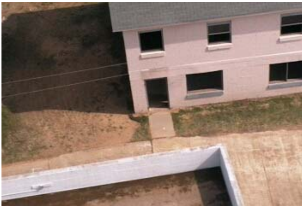
Fig. 7. Camera placed with selected building opening in center, in this case an open
