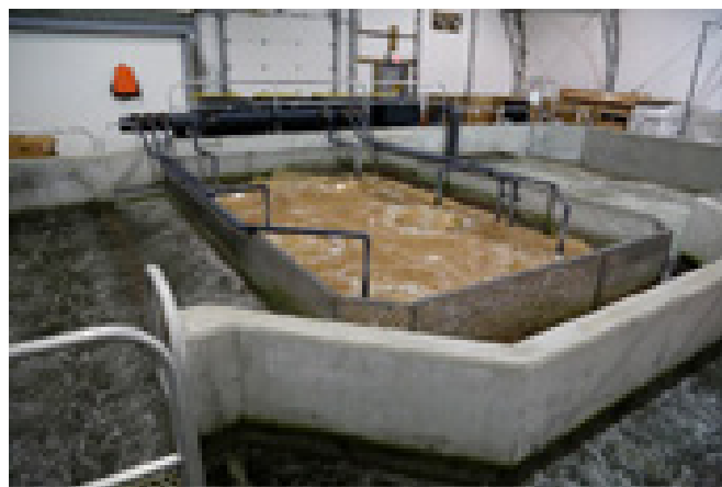
Figur 7.5. Biofilter (Inter Aqua Advance) ved Marine Harvest Canada.
