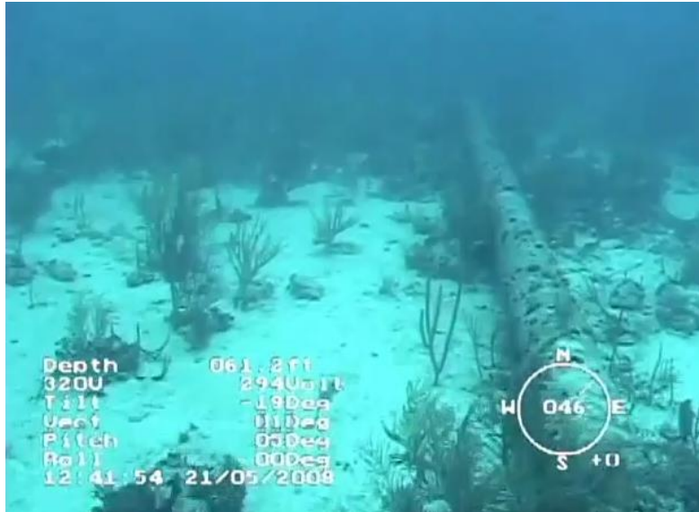
Pipeline inspection with a Remotely operated vehicle (ROV)
