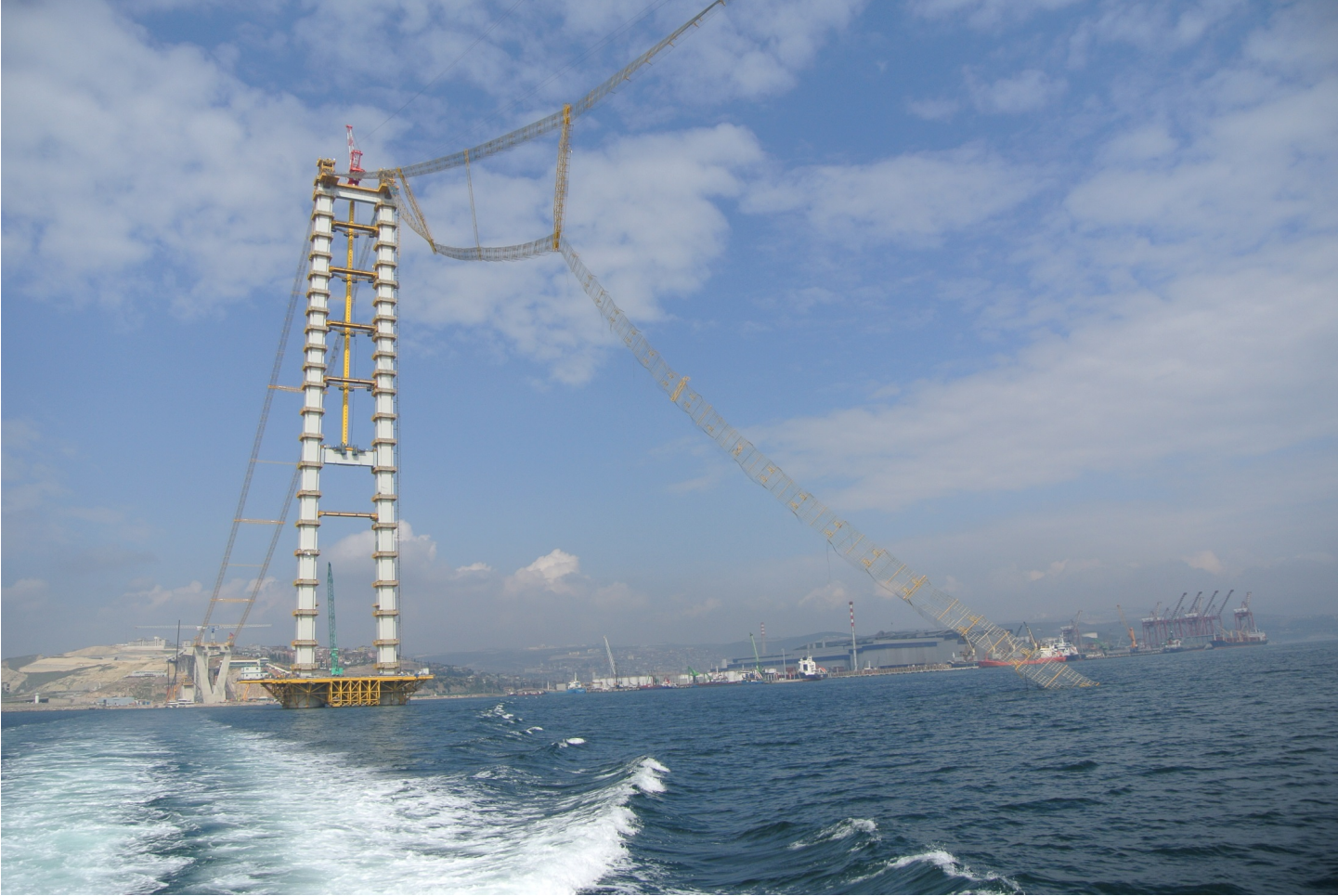
Rare Events: Collapse of Cat Walk in extreme Wind Regime
