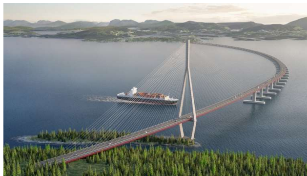
Fig. 1 Artist impression of an "early phase" floating bridge for Bjørnafjorden, Norway.
