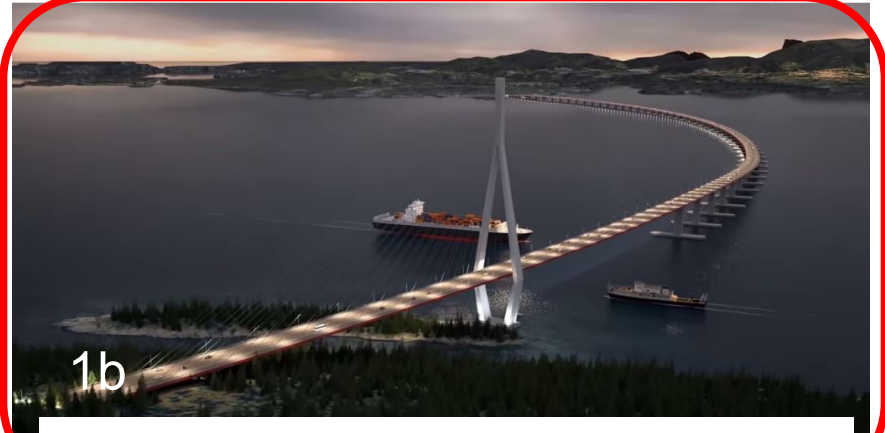
Bjørnafjorden bridge (≈ 5 km)
