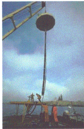
Photo: Technocean, Gothenburg, Sweden, 1984
