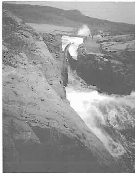
Figure 2. Wave increasing in amplitude as it propagates in the rock-blasted wave collector before entering the narrower energy-converting channel.
