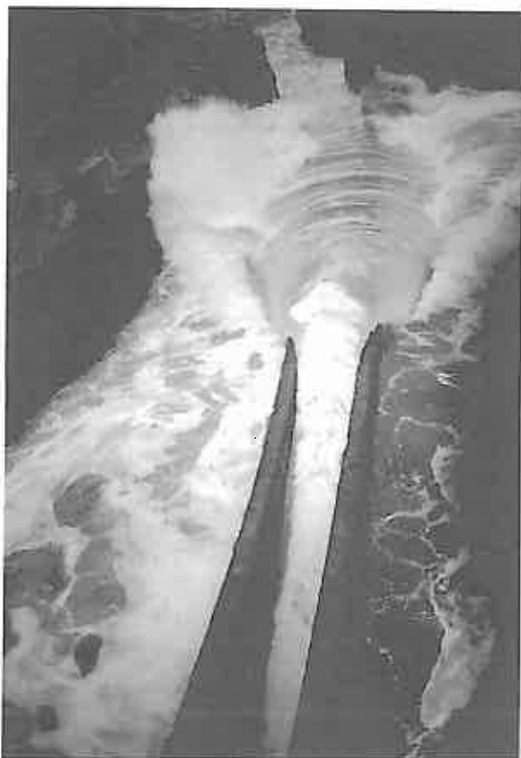
Figure 3. Wave crest spilling over the concrete wall of the tapered channel and into the water reservoir.
