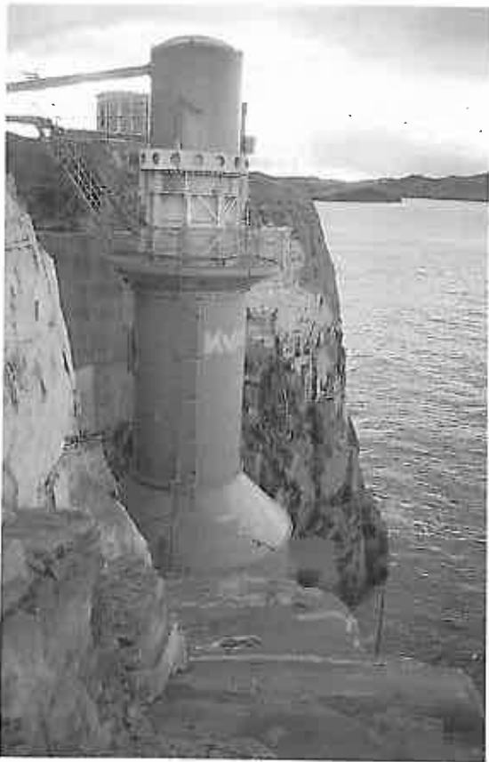
Figure 7. The Kvaerner OWC wave power plant constructed in a steep shore cliff at Toftestallen.
