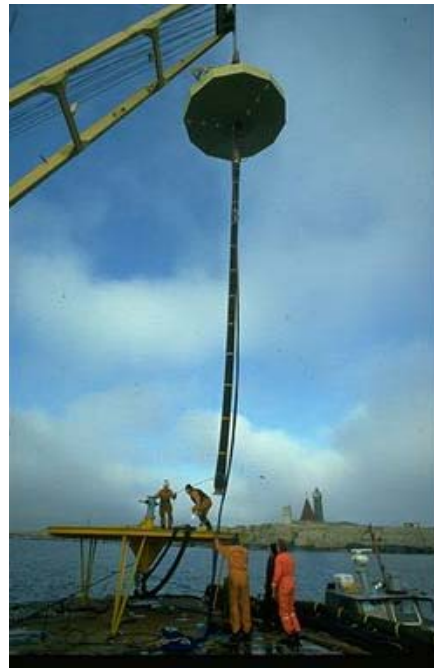
Photo: Technocean, Gothenburg, Sweden, 1984
