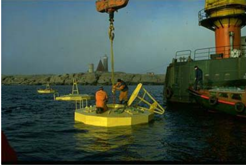
Photo: Technocean, Gothenburg, Sweden, 1984
