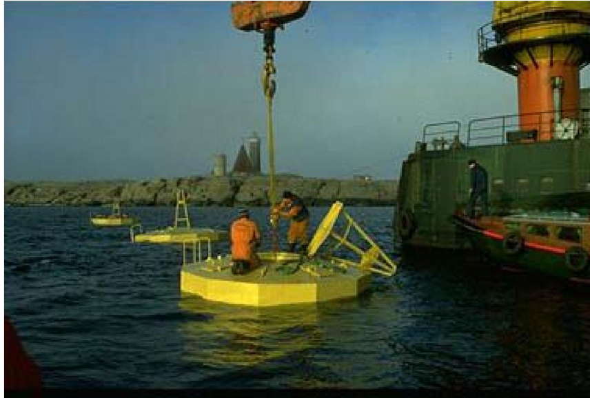
Photo: Technocean, Gothenburg, Sweden, 1984
