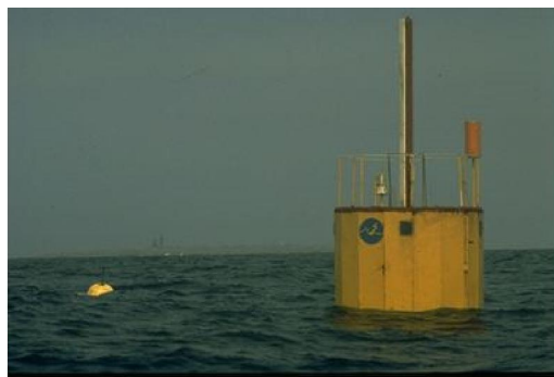
Photo: Technocean, Gothenburg, Sweden, 1981
