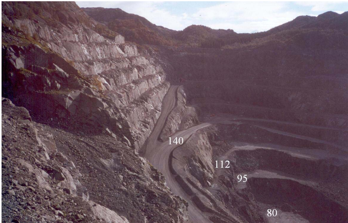
Figure 7. The footwall at the Eastern part of Tellnes open pit mine as seen in October 2002. The main transport road is at level 140 and the bottom of the pit at level 80.
