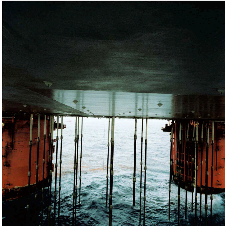
Figure 10.9: The wellbay on the Snorre TLP ( www.statoil.com ).
